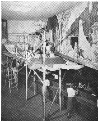
The fresco in progress showing wall curvature at top, left
